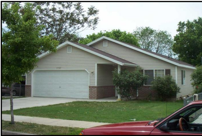
Picture 9 - New Construction one story housing style
