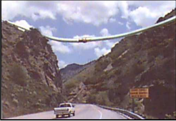
Picture 8 - An artist's concept of using the existing water pipe as a gateway into Ogden Canyon
