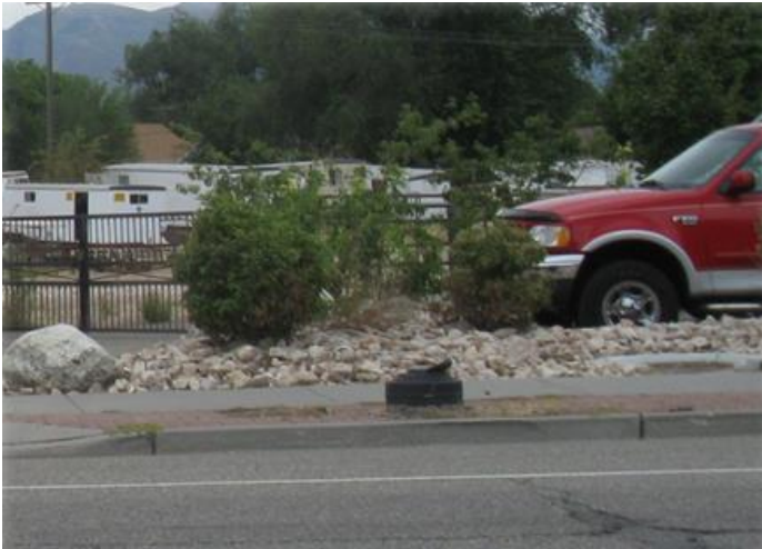
Repair and Replace Damage Features along 24 th Street
