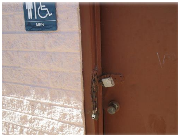
Improve Access to Park Restrooms
