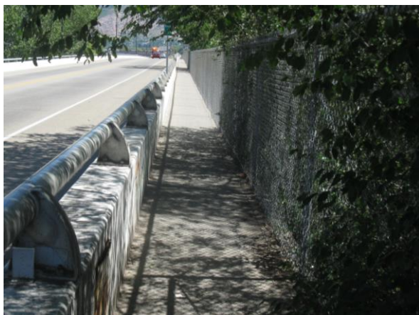
24 th Street Rail-Yard Bridge Sidewalk
