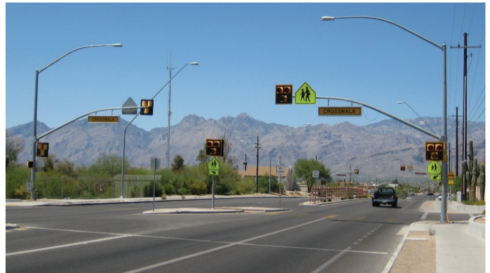
Below: Example of Recommendations (overhead HAWK beacon, center pedestrian refuge, and intersection lighting)
