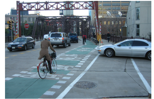
Above: example of bike lane with green intersection highlights
